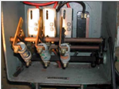
Fuse box/switch gear, fuse shields/flash guards – asbestos cement
