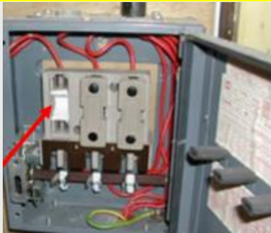
Fuse box/switch gear, fuse shields/flash guards – asbestos cement
